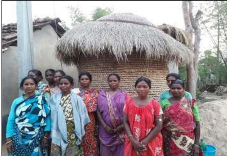
A well-built community grain store locally called 'Gola ghar' was constructed with the full participation of all group members. DRCSC helped the group by providing the expenses for making the cement floor. It was made sure that the stored grain was kept dry and free of pests by constructing the store in a well lit place and making a thatched roof. The preliminary grain collection of 100 kg was shared equally by DRCSC and community members.
